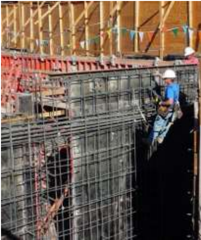
4. Reinforcing steel for concrete wall construction. (Schexnayder)
