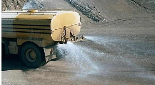
Figure 5. Water truck adds water to a fill.
