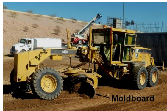
Figure 10. Grader finishing a fill.
