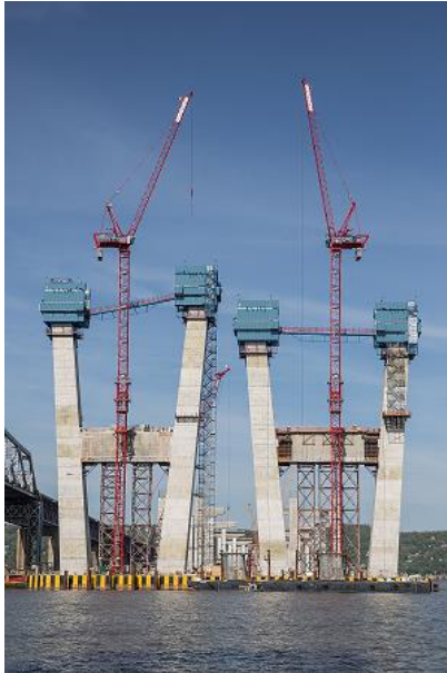
Figure 5 - Jump form tower construction in progress
