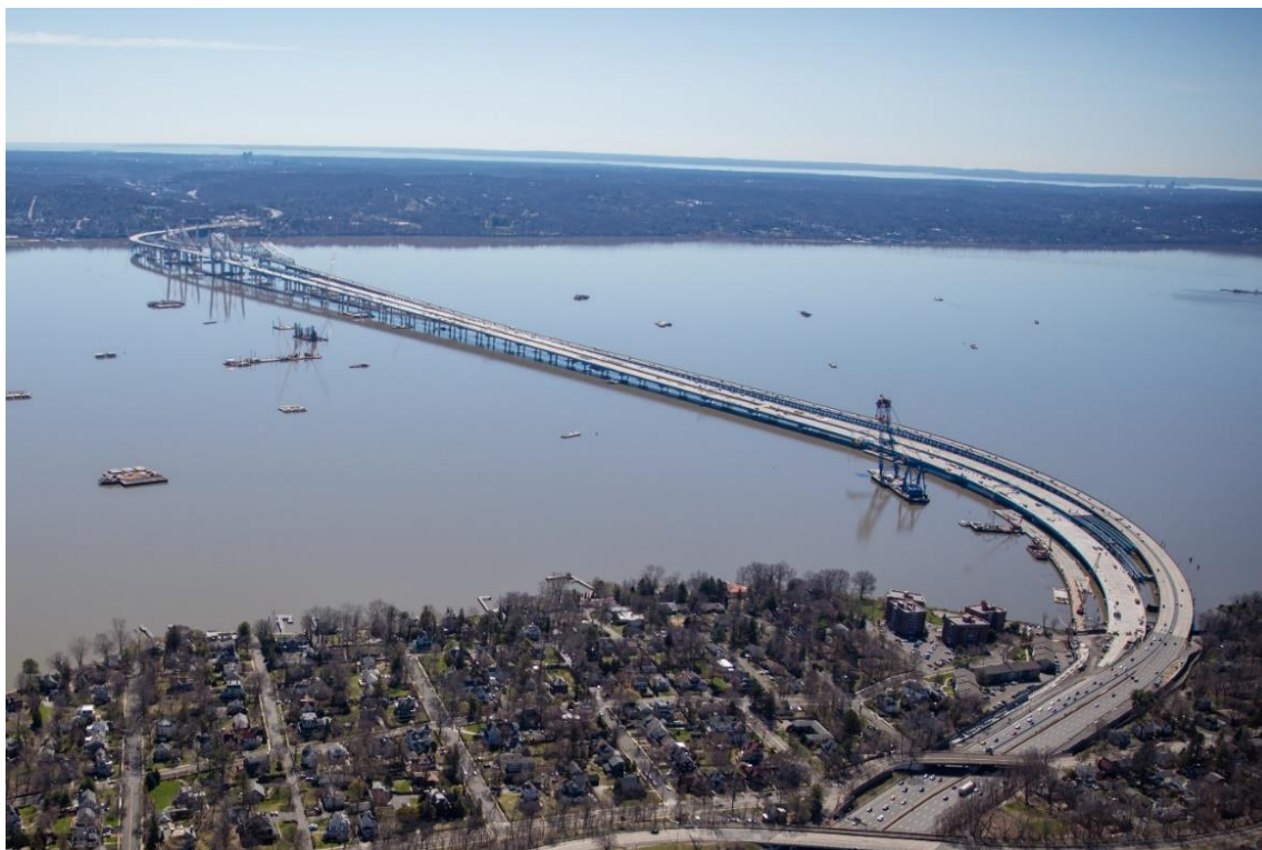
Figure 1 – General view of the Rockland Approach of the Governor Mario M. Cuomo Bridge over the Hudson River, NY
