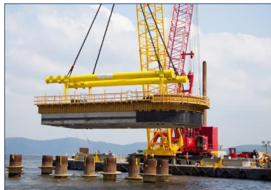
Figure 4 - Setting a precast pile cap "tub"
